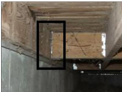
7.4 Picture 1 Missing Joist Hanger
